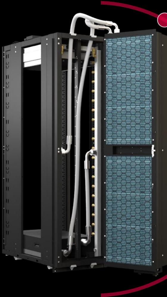
Installation frame for routing the hoses
